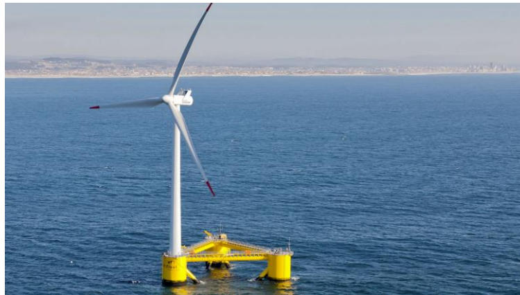
Figure 79: Principle Power WindFloat Atlantic Semi-Sub [56]
