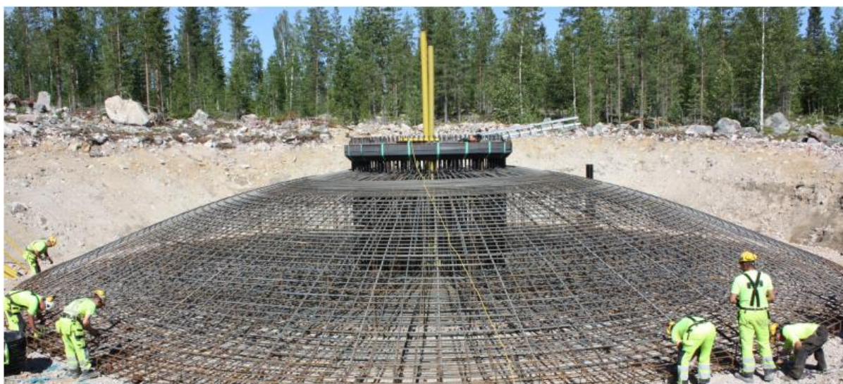
Figure 66: Onshore Wind Foundation: Reinforced Concrete Gravity Base (Image Courtesy Ramboll)
