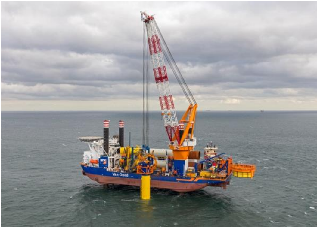
Figure 72: Jack-Up-Barge installation of Monopile - Credit: Van Oord
