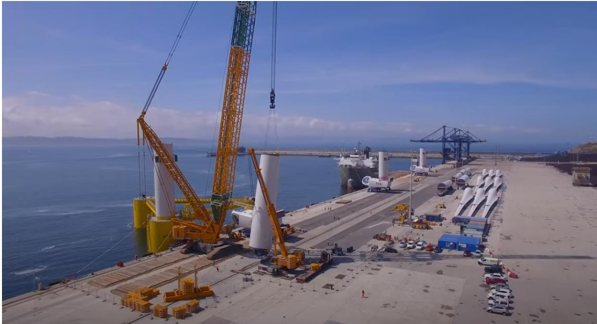
Figure 58: Turbine Tower Assembly for FOW
